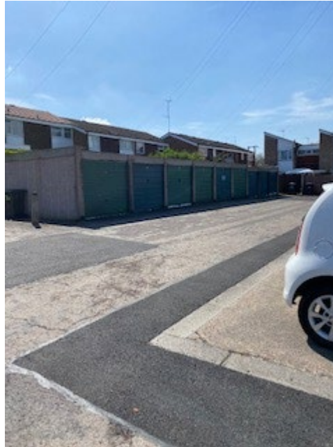
Garages to be demolished the south west
