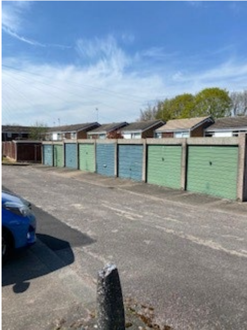
Garages to be demolished to the north
