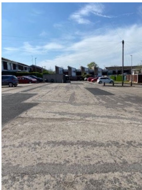
View across parking
